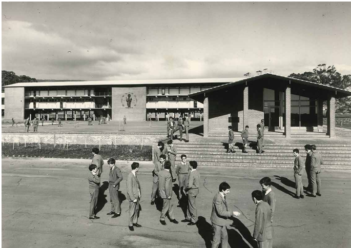
FIRST SENIOR SCHOOL BUILDINGS - ADMIN & CLASSROOM BLOCK
