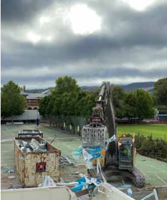
DEMOLITION FOR THE MARY GLOWREY CENTRE BEGINS (JS)
